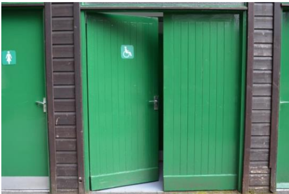
Above: Accessible toilet outside the visitor centre
